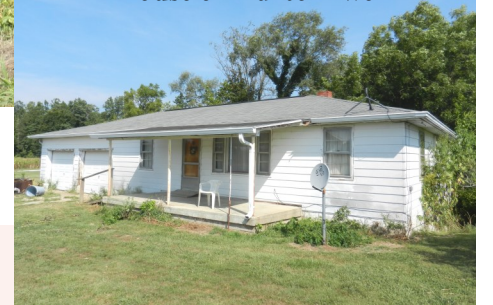
House on Parcel Two
